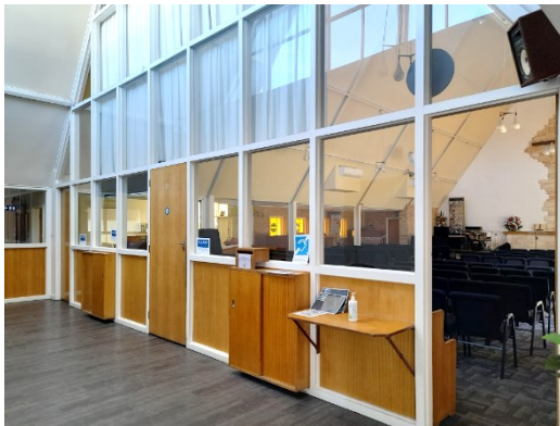
Glazed partition wall between foyer and chapel
