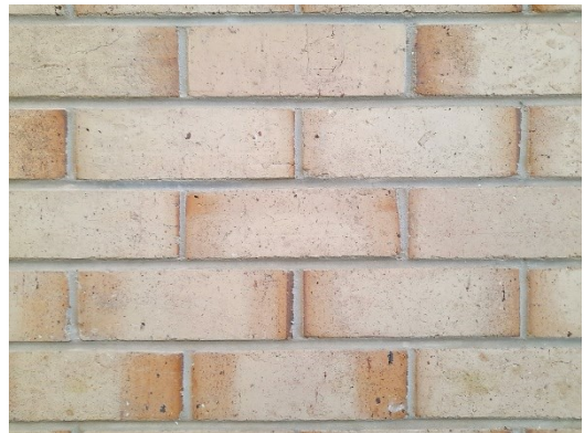
Face brick in chapel
