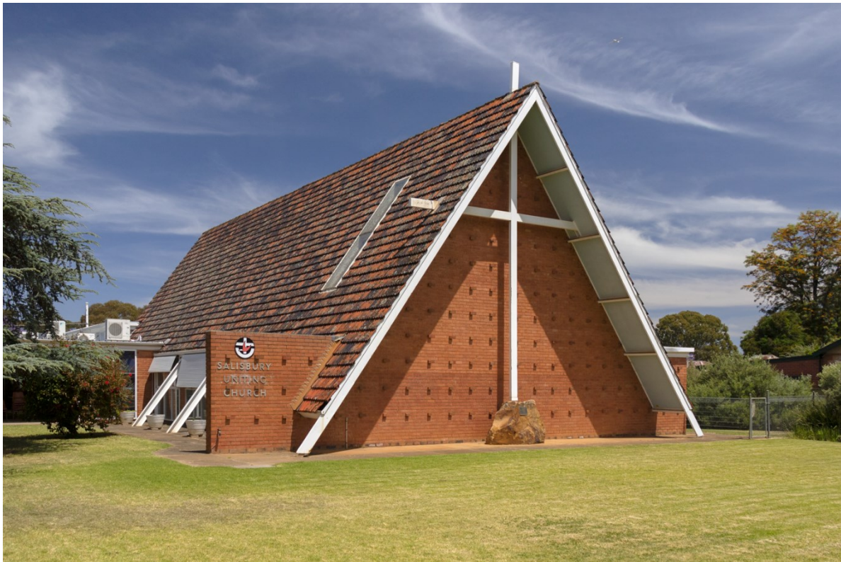
Former Salisbury Methodist Church, 2 November 2023
