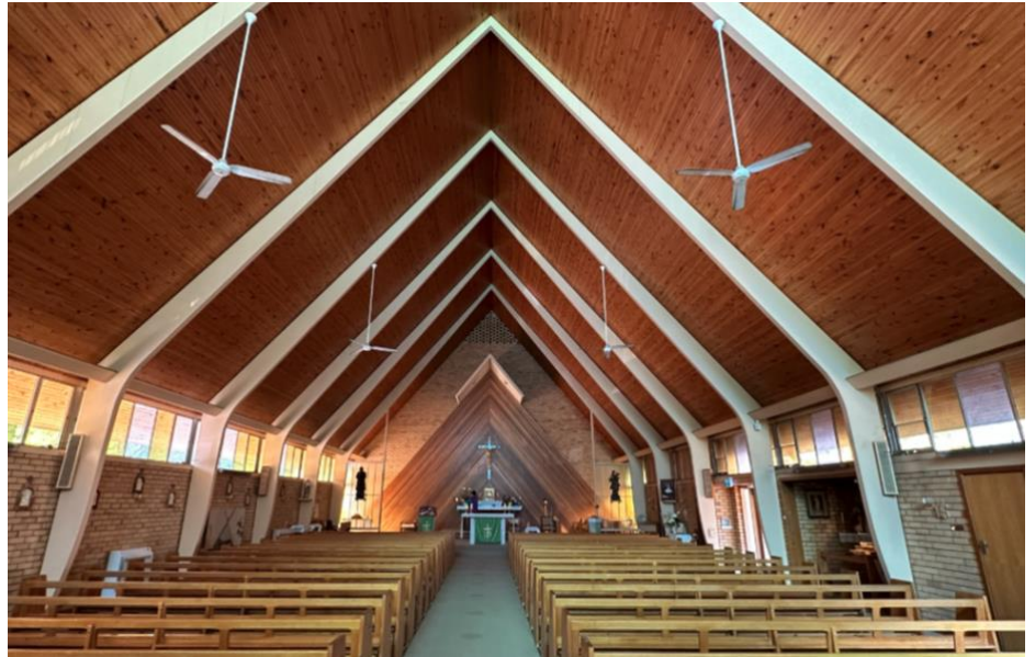
Image 3. St John Vianney's Catholic Church interior with clear spanning steel portals.
