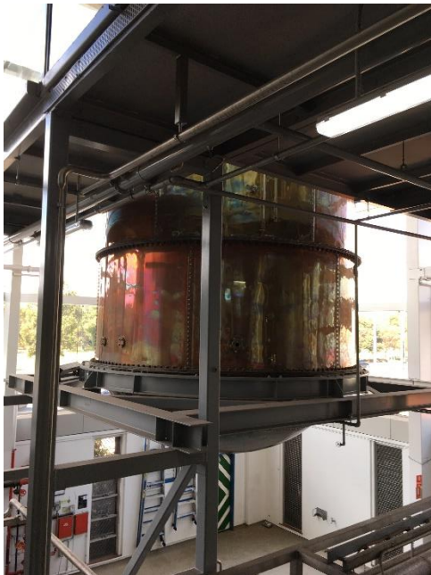
Copper kettle, showing riveting and rounded base.
