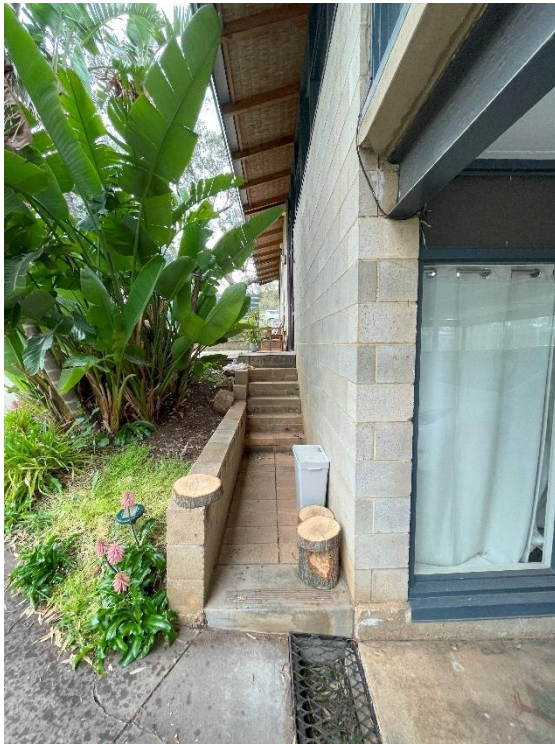
Concrete pathway, fence and stairs
