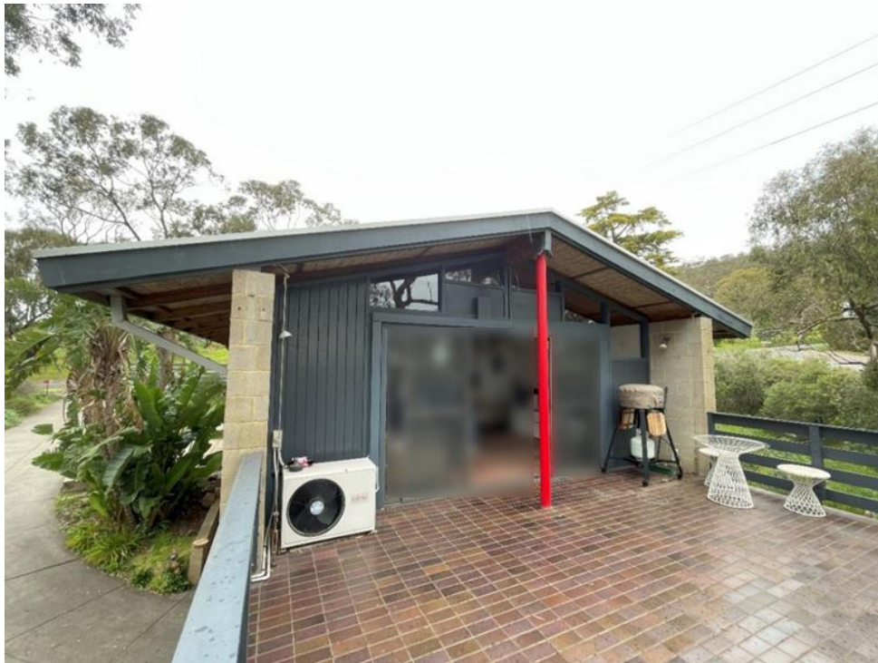
Western elevation showing balcony extension (upper floor).
