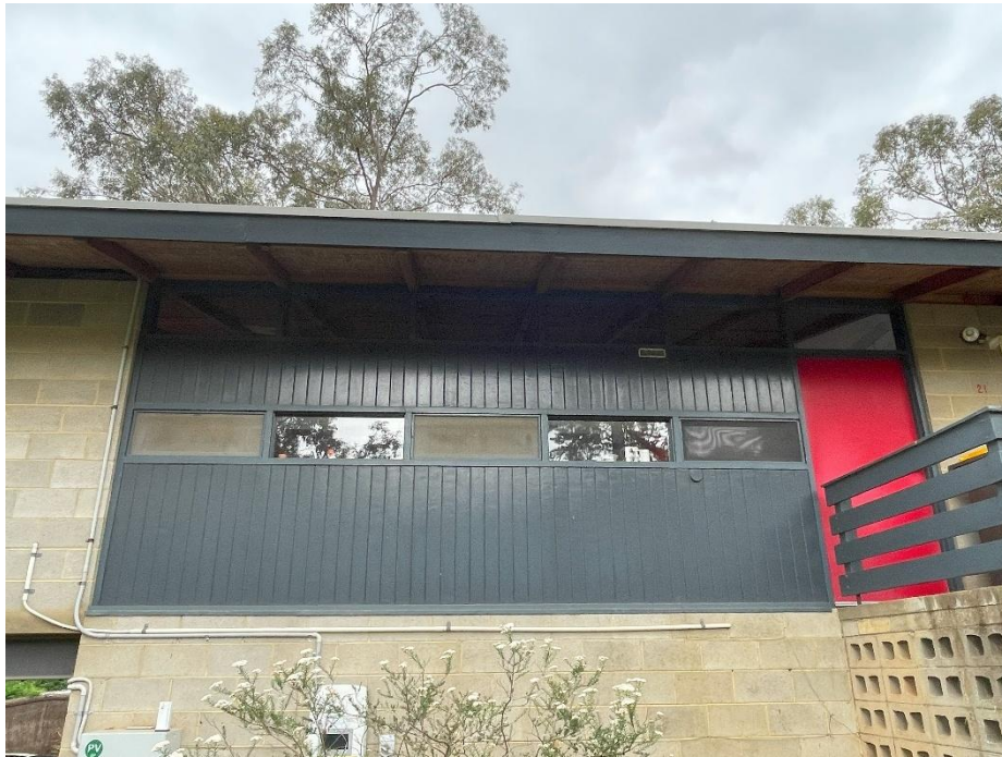
Corbusian-inspired window pattern on southern elevation (non-original paint); exposed perforated Besser blocks can be seen to the right.
