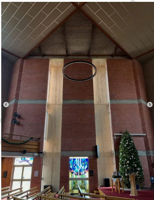
Internal northern elevation.
