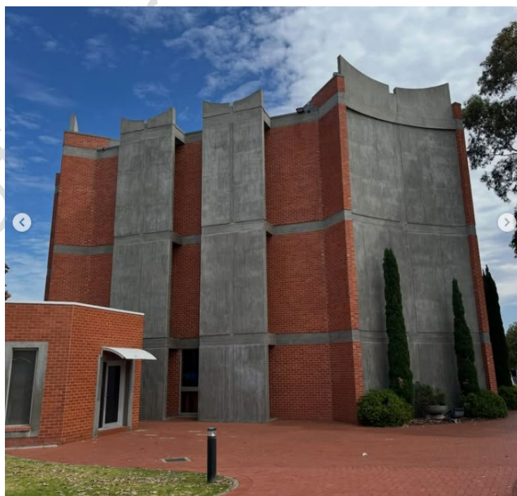
Exterior showing southern and southeastern elevations.
