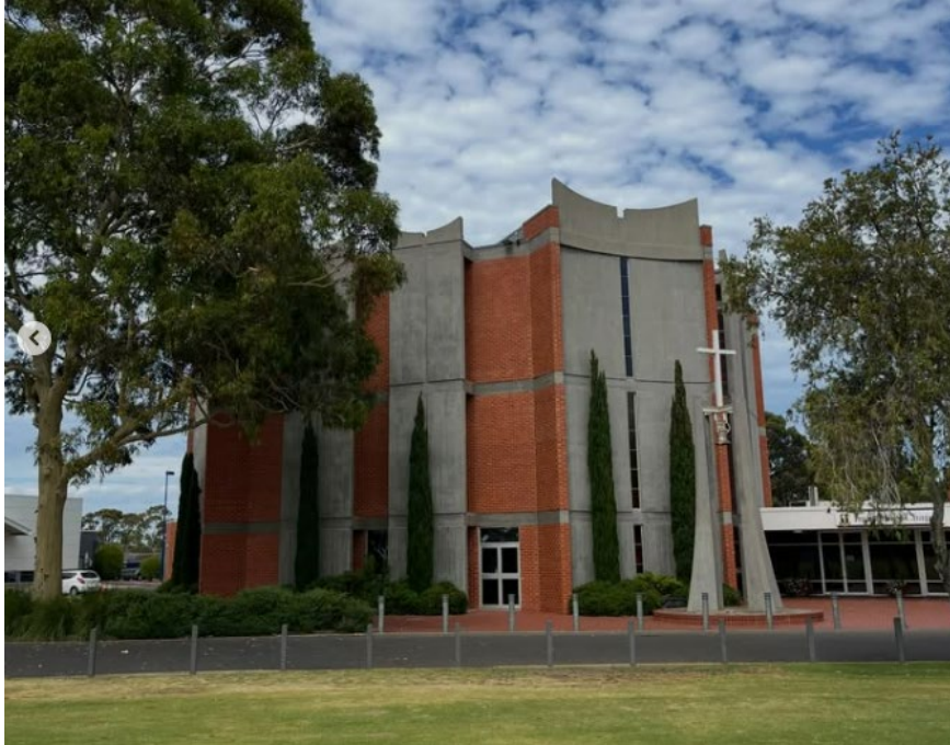
Exterior view showing eastern and northeastern elevations, note relocated belfry on right.
