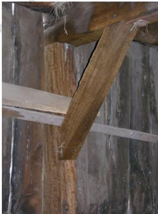
Detail of Barn 1 interior.
