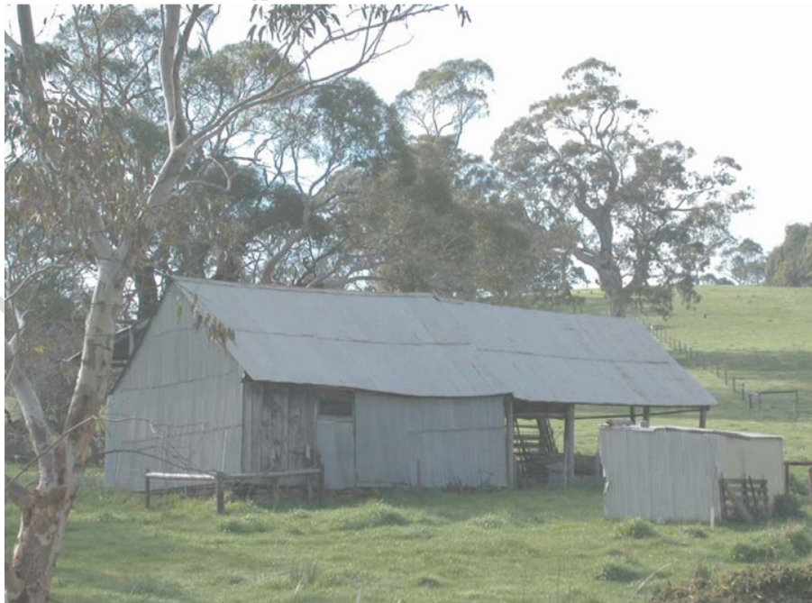
North-west elevation of Barn 2, note the timber slab to the left of the building.
