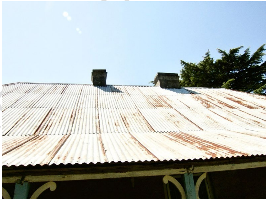
Two chimneys, the larger of which is a part of the loft smokehouse.
