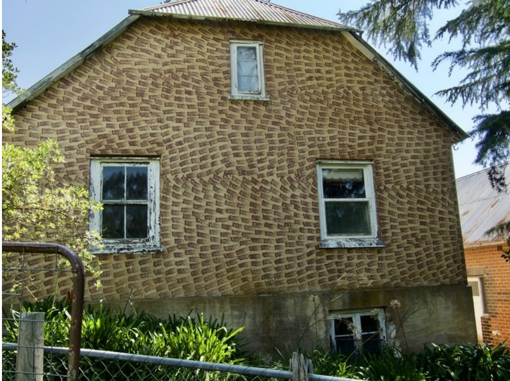
Eastern elevation of the farmhouse, 2021. Note gable end loft window.
