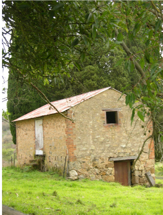
Stone outbuilding, note the timber lintels and red brick quoining.
