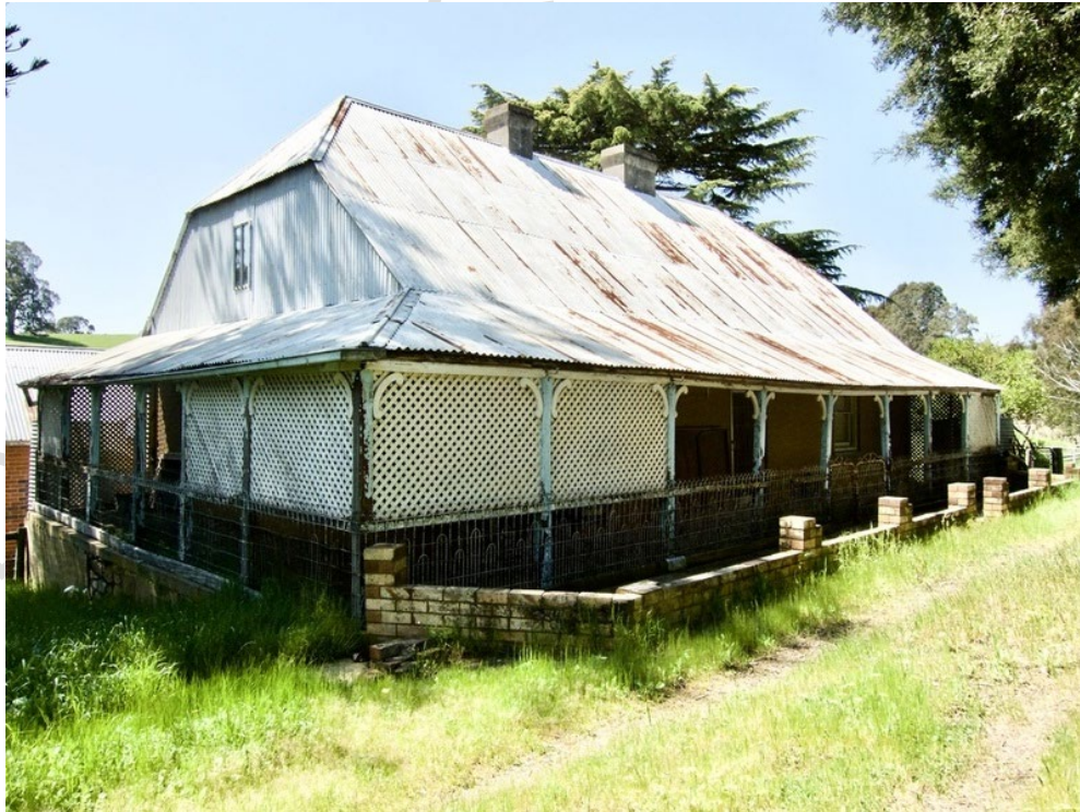
South-west elevation of farmhouse, 2021. Note the half-hipped roof with corrugated galvanised iron covering timber-shingle roof, the twin chimneys and the gable end loft window.
