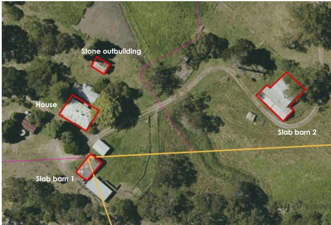
Former JF Paech Farm Complex, Paechtown SA; CT 6249/253 D124371 A100; CT 6249/254 D124371 A101; CT/5494/892 F7975 A1; CT/5085/934 F7975 A2 Hundred of Kuitpo.
