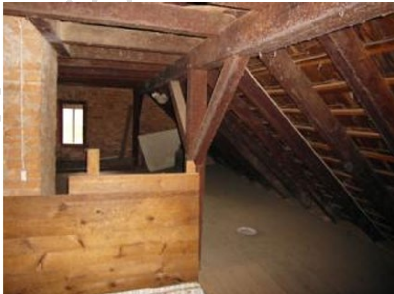
Smokehouse in farmhouse loft. Note the red gum timber frames and stringy bark shingles.
