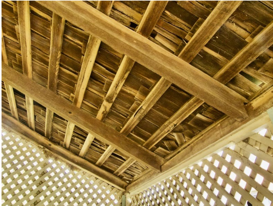
Original stringy bark roof shingles.
