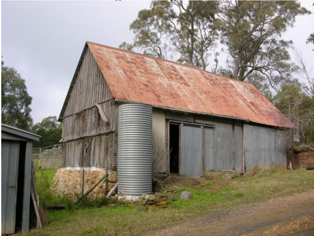
Northern elevation of Barn 1.
