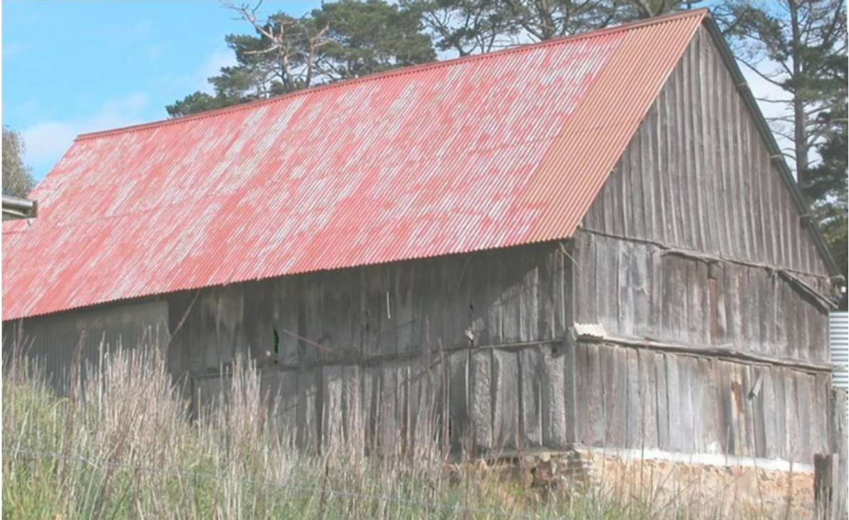
Slab Barn 1 from north-east elevation, 2004.
