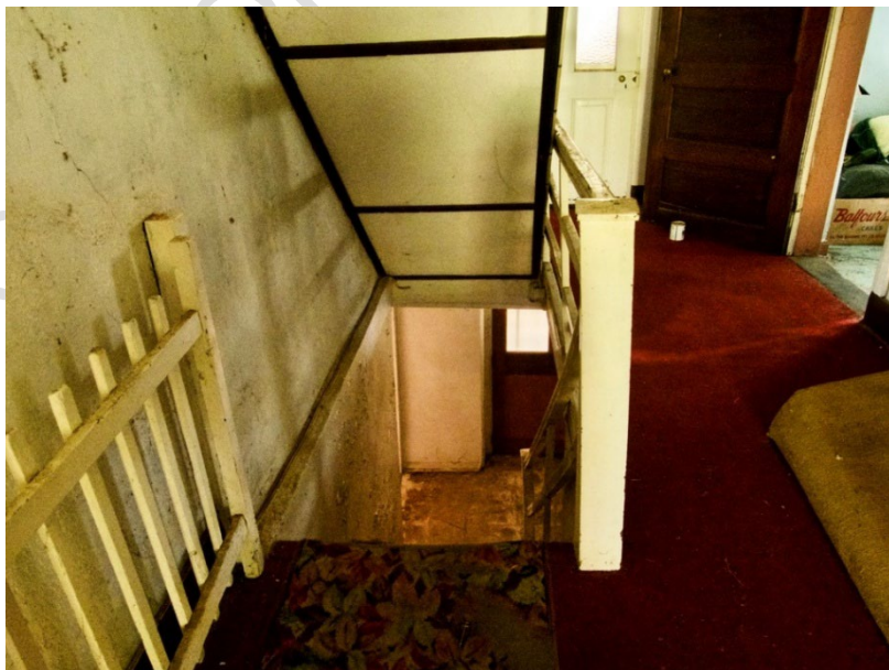
Interior of house.
