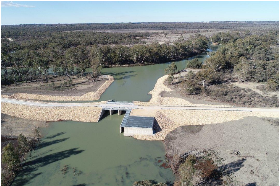
Figure 1. Katarapko regulator and fishway built as part of SARFIIP
