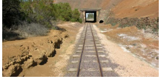
Moonta Mines mining infrastructure, railway DEW 2022
