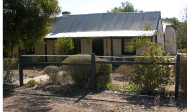
Moonta Mines, vertical proportioned openings. DEW 2022
