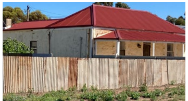
Moonta Mines, cottage, timber framed verandah, DEW 2022
