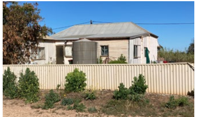
Moonta Mines, cottage, lean to addition, DEW 2022
