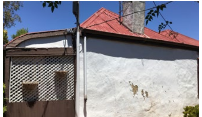
Moonta Mines, cottage, double hipped roofs, DEW 2016
