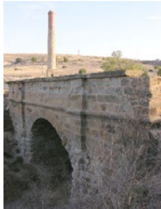
Mine Bridge DEW 2005
