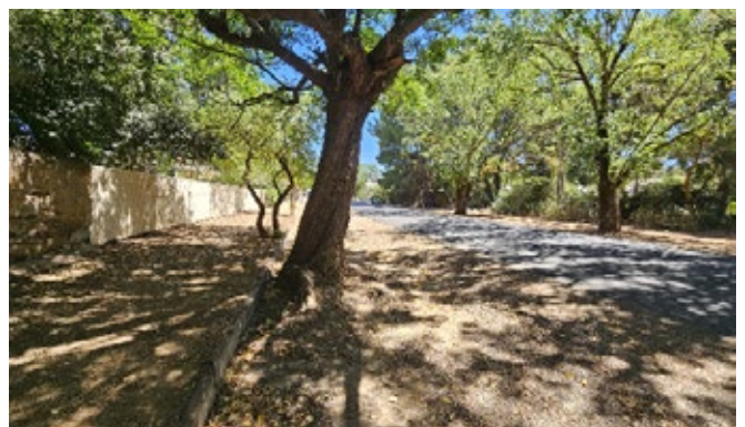
Bluestone kerb, wide informal verge and unsealed footpath, Chapel Street DEW 2024
