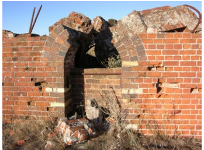
Burra Mines smelter chimney remnants. DEW 2005
