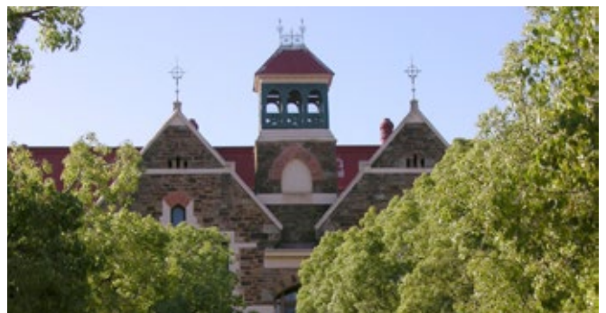
Above: St Mary's Anglican Church, Market Street DEW 2016
