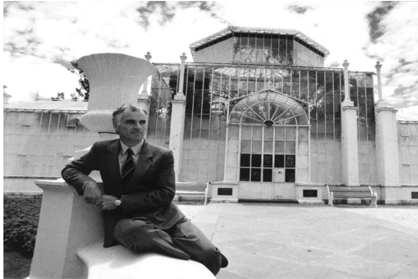
Figure 2.24 A dilapidated Palm House, prior to restoration, with Dr Brian Morley in the foreground.
