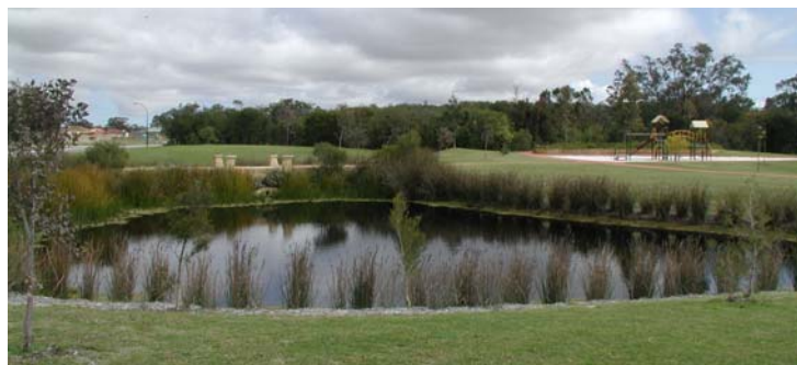
Figure 10 Example of an earthen sediment basin with edge vegetation
