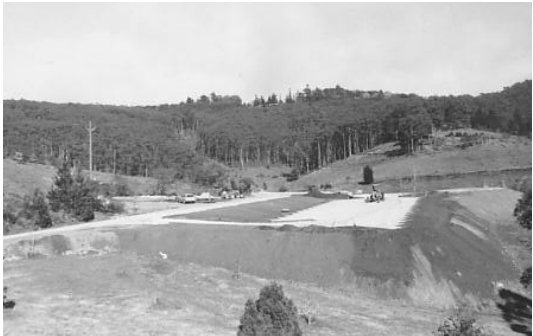
Figure 2.1 Photo: Construction of the Lower Car Park in 1977. Source: Noel Lothian.
